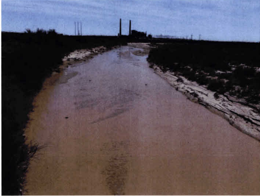
Photo #1: Cholla Power Plant and Little Colorado River from Obed Road Bridge
